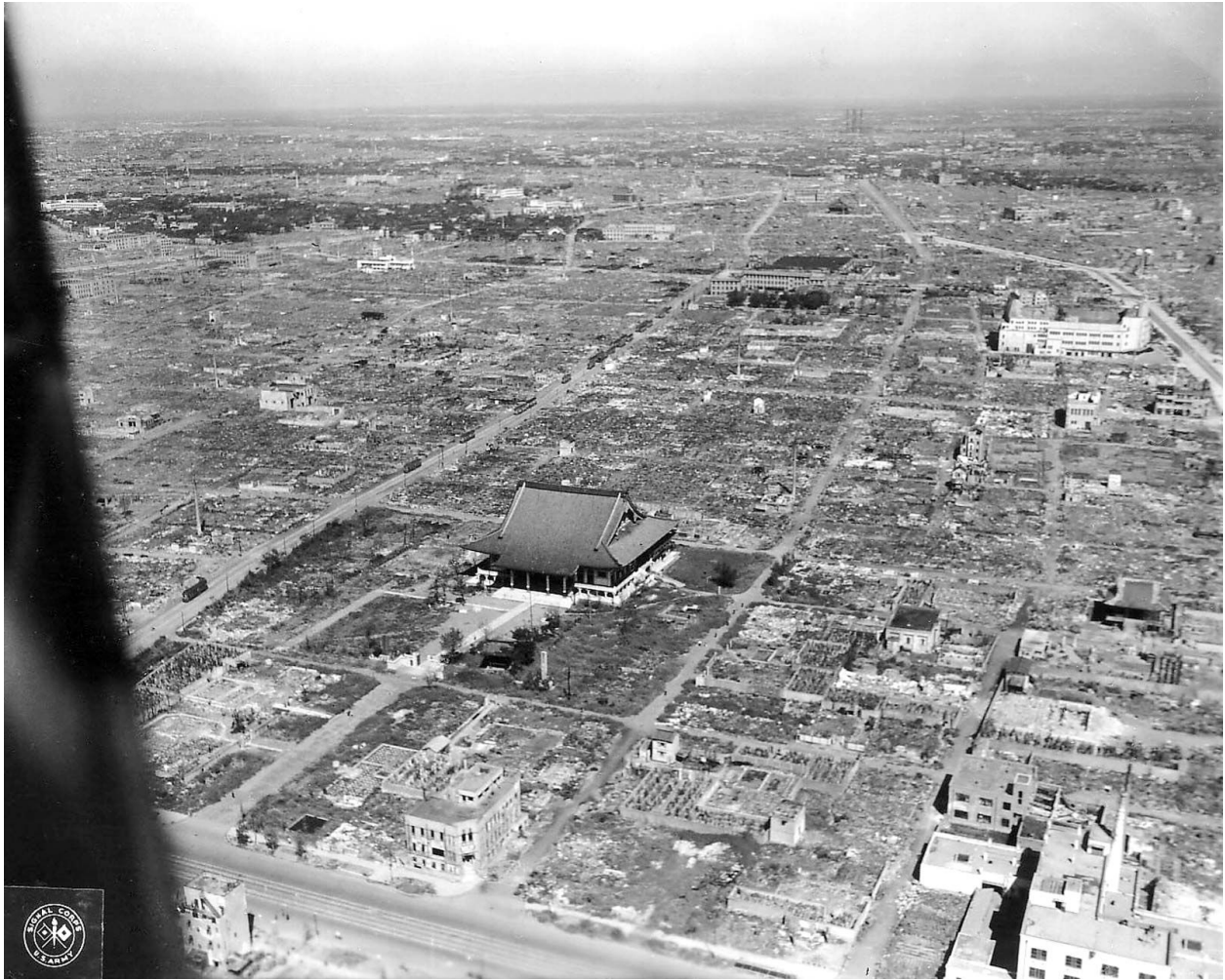
Massive damage from firebombing of Tokyo
